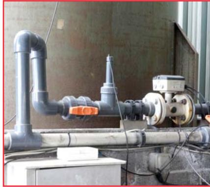
Typical installation of our PES2-QR inline pH electrode system with quick release fitting, where the pipework cannot easily be drained for calibration.
